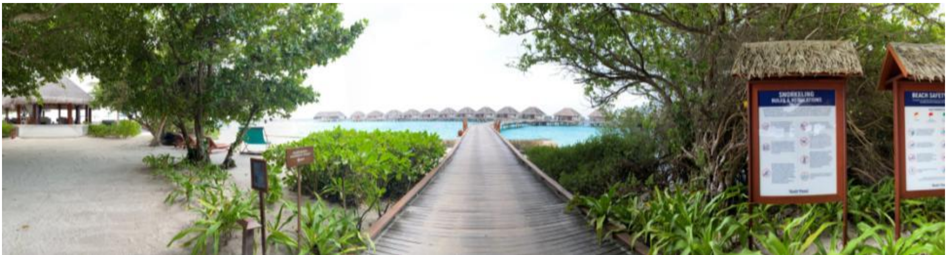
VIEW OF THE SUBJECT PROPERTY: A HOTEL NAMED “DUSIT THANI MALDIVES” - (PHOTO VIEW POINT NO. 5 AND 6)
